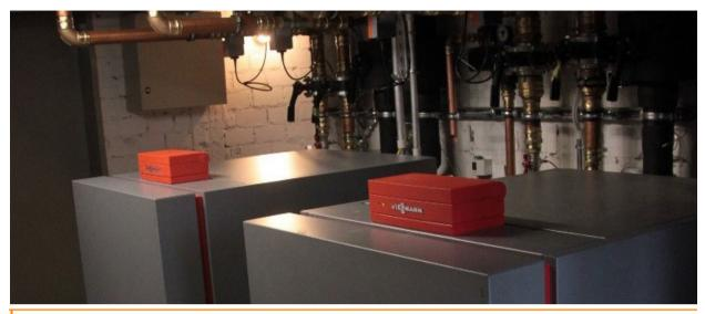
The heat pump hydraulics of the HEAVEN system exploits the synergies of air (availability, cost) and geothermal energy (temperatures, efficiency) and solves the problem of limited space in cities.
